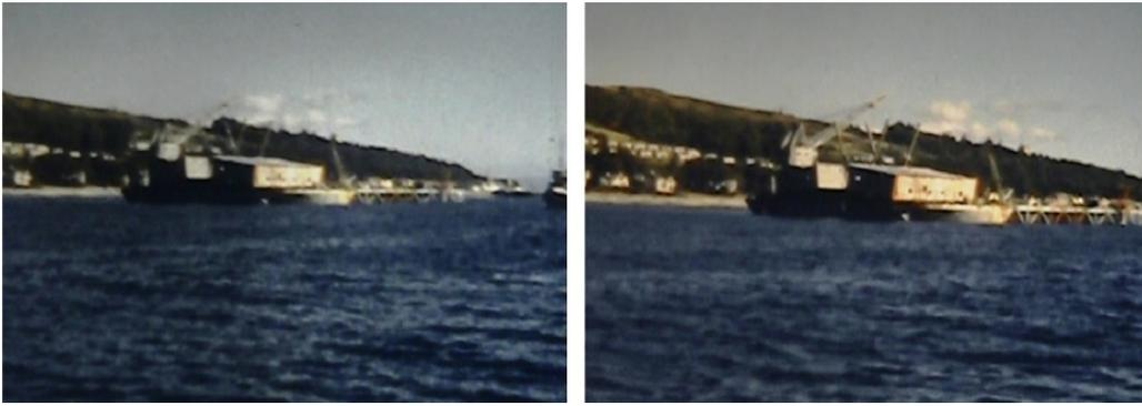
These color pictures were taken with my Bell & Howell 8 MM movie camera as a crane was being transferred to the top of wing walls A and B. Note the gantry structure at water level in the picture on the right and the crane at the back of section C. I had the 2 & 3/4 inch reels of film converted to a DVD & received several of the pictures as still images like these. All my color pictures are from the 8 MM film.
